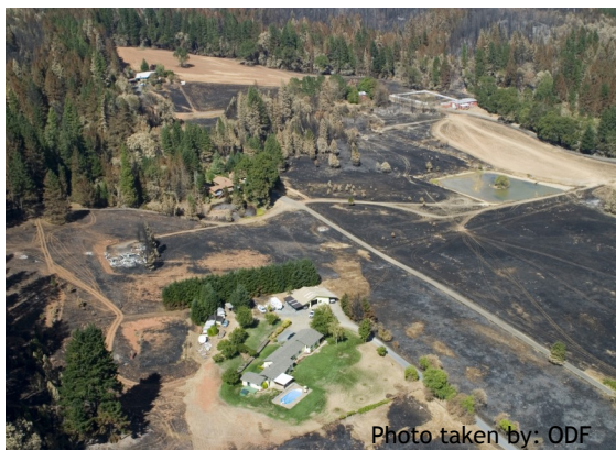
This photo elaborates on how the fire moved through brush and towards a housing community. This hillside home in Ashland had a defensible space around it. The Siskiyou Fire was traveling in the crowns of the trees rapidly up the hill towards the home. This photo was taken literally moments after the fire hit the thinned defensible space area and died down to nothing.
